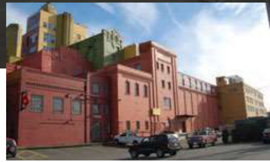
Rainier Commons: PCB-laden paint
