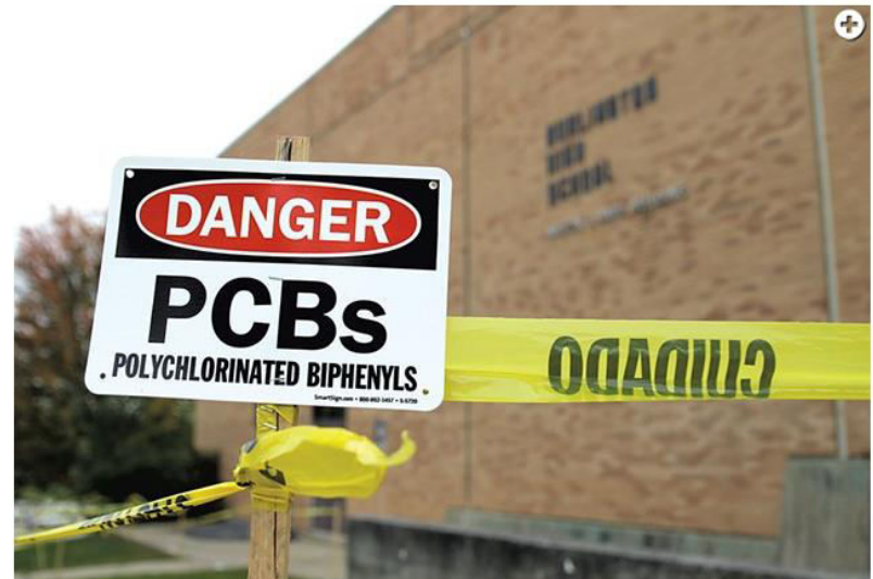
Signs warning about PCBs at Burlington High School
